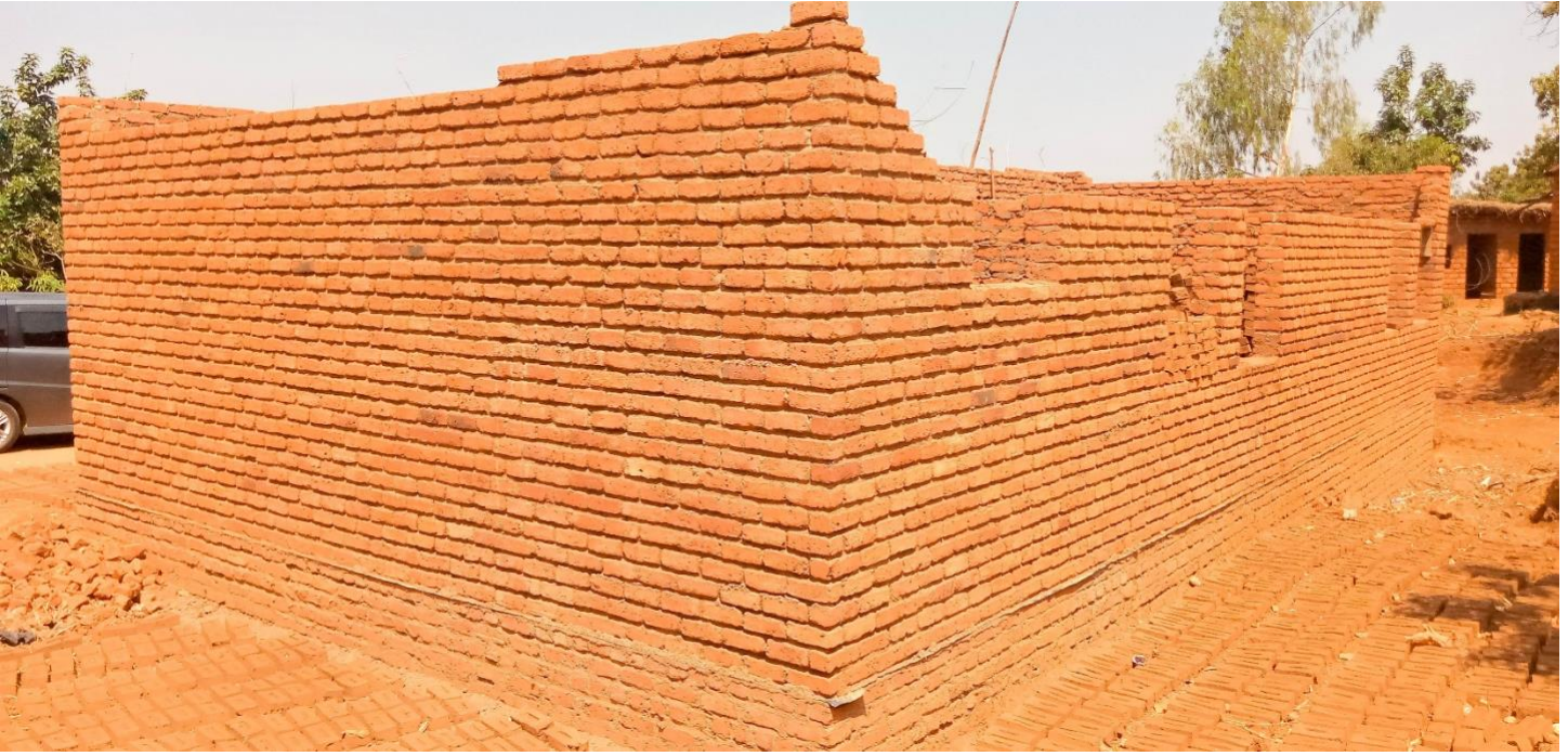
Left rear angle view of the building.
